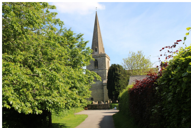
St Peter's Church, 900 years old this year and a Grade 1 Listed Building within Cassington's Conservation Area.
