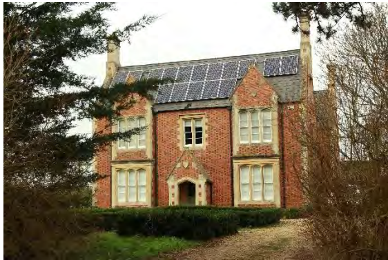
Manor Farmhouse Notable 19th century building (formerly Cassington House). Red brick building with stone quins (often used to reflect higher status buildings) of two storeys with attics and a slate roof.
