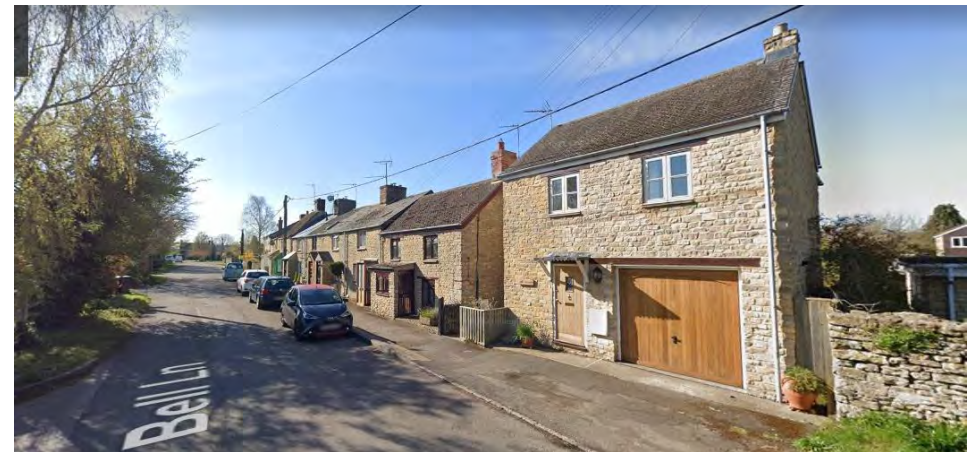
Terrace in Bell Lane including a later addition of Lilly Lodge as an excellent example of the use of traditional detailing © Google 2021
