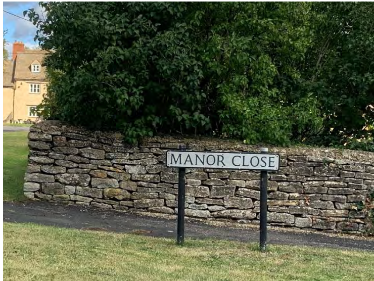
Drystone wall at Manor Close with the Chequers Inn terminating views into the Conservation Area party seen in the background
