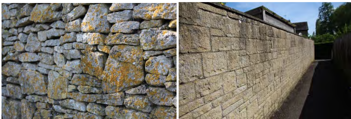
Figure 27. The strong contrast in construction and wildlife friendliness of old dry stone walls compared to modern built stone walls in Cassington. Both photos from the vicinity of the foot path from the Upper Green to the Lower Green. The old walls have many living spaces for insects, slow worms and other organisms and a strong growth of lichens.
