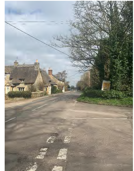
Grade II listed The Laurels with Significant Trees on eastern boundary of Yarnton Road
