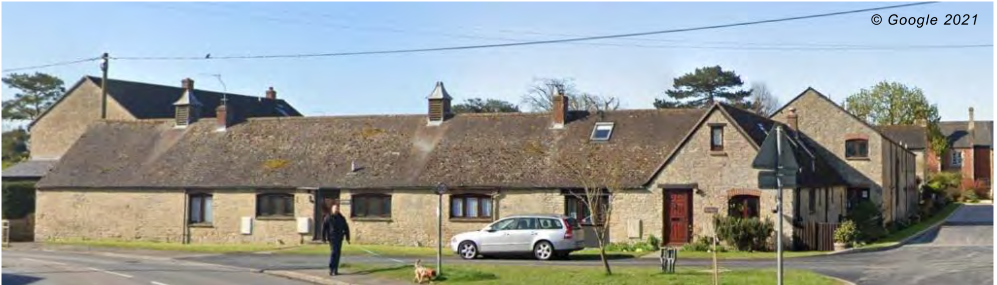
4-8 Hollow Furlong, Wild Forest and The Old Stables Former barn buildings converted as part of cul-de-sac development in 1980s.
