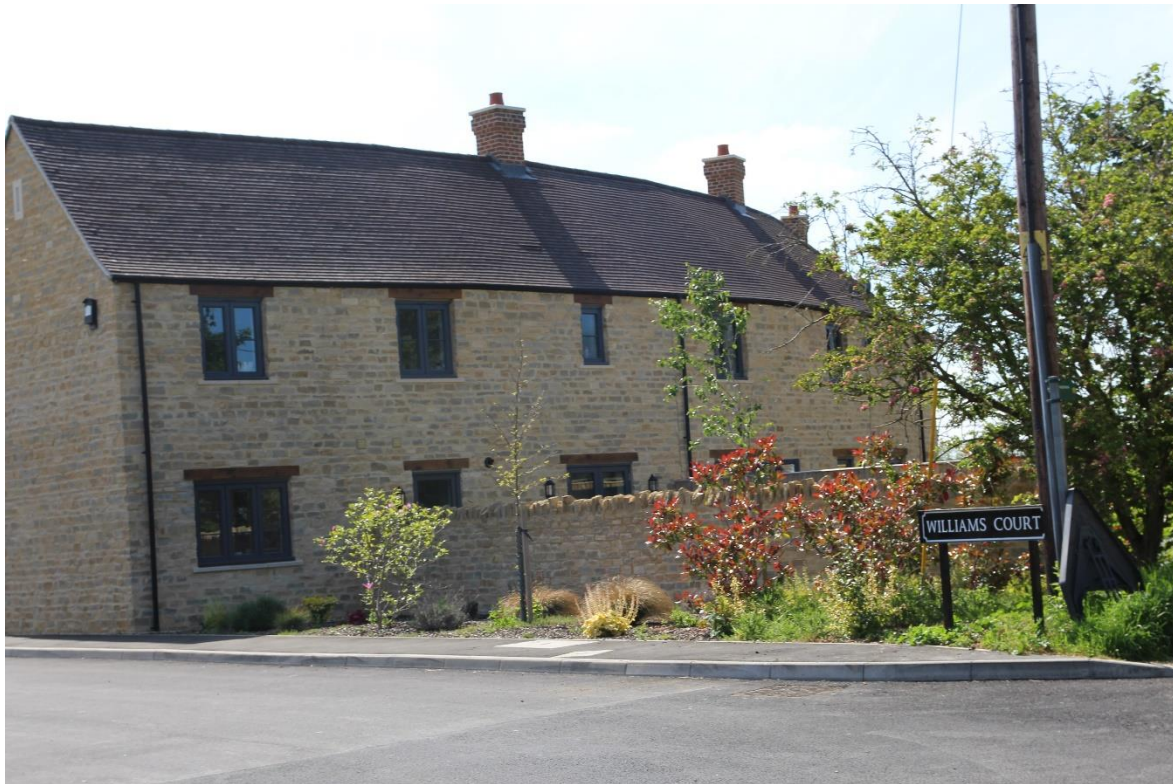
Figure 17. Recent development off the Upper Green at Williams Court. Note that although the stonework is similar to the “ideal” development in Figure 16 the roofing material is modern and not in keeping with older buildings.
